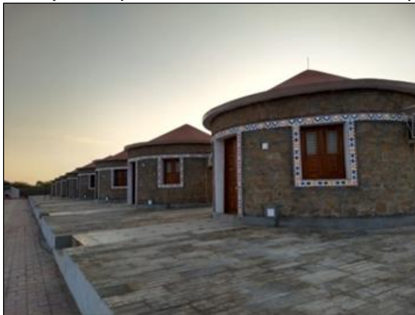
Fig. 5: Bhunga connected through plinth
