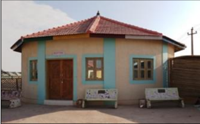
Fig. 10: Roof constructed with Mangalore tiles
