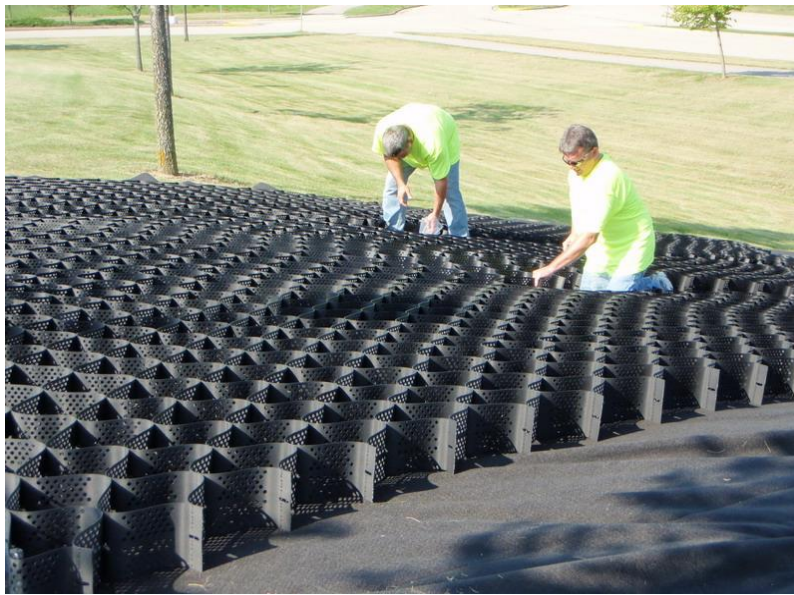
Fig. 1: typical geocell
