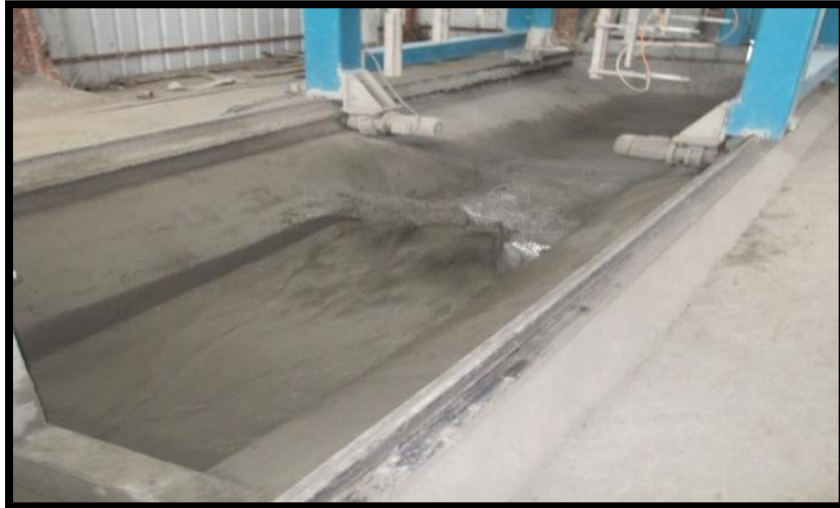
Fig. 4: Waste Slurry Tank
