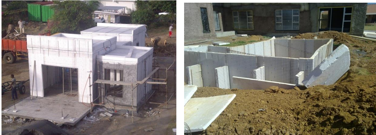
Fig. 7 & 8: Reinforced EPS: “Thermally efficient construction”
