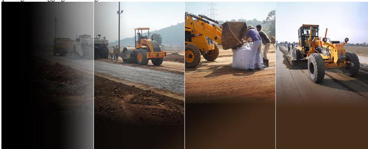
Fig. 15 & 16: Global road stabilizers: “For roads that are ‘Hard’ to beat”
